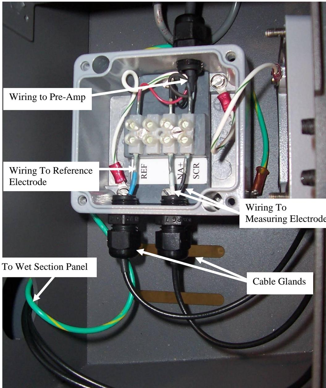
**Figure 8.** Sensor wiring to the junction box.
